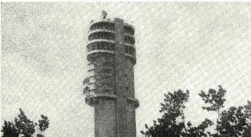
Below: View of the 300' microwave tower recently completed for the Federal Telecommunication Laboratories at Nutley, N. J. The tower houses experimental antennas and equipment for research and development work in television, aviation communications, multiplexing, microwave antennas, point-to-point communications, etc. Right: Three-bay RCA super turnstile tv antenna being mounted atop an RCA pylon i-m antenna for WBZ-TV near Harvard Stadium, Mass. Tower is 656' high and designed to service an area of 40 miles radius of Boston.
